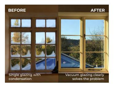
Vacuum Glazing is highly efficient double glazing. Like standard double glazing, it is made with two panes of glass separated by a cavity. However, instead of the usual gas or airfilled cavity, all air is extracted, and the unit is completely sealed.
